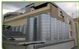
Cylindrical silencers with and without nucleus
